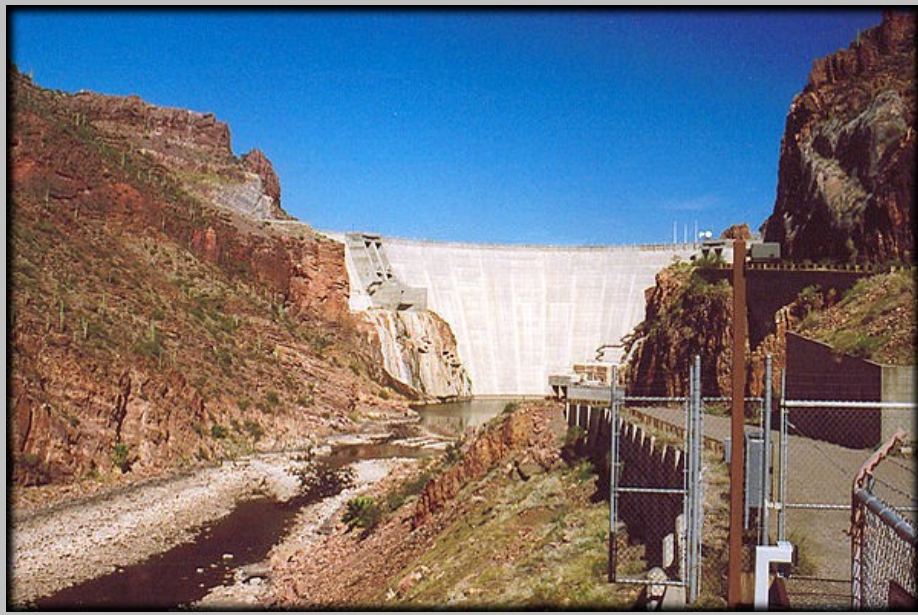
The “new” Roosevelt Dam, looking upstream from the Salt River bed, along the Apache Trail (SR88), in the Superstition Mountains of Arizona.
